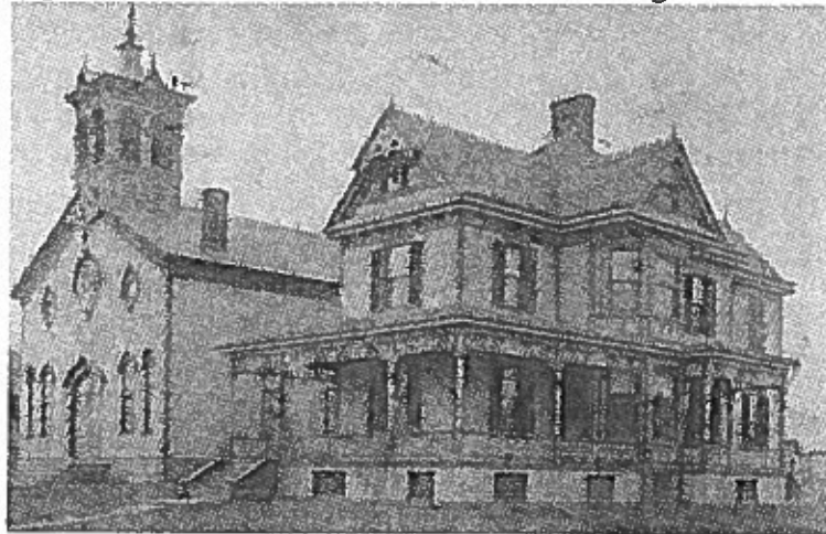
Figure 21: Methodist Church and Parsonage
