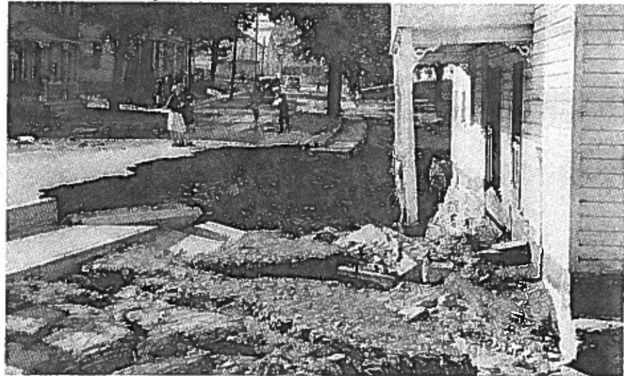
Figure 34: Prospect Avenue after the Flood
