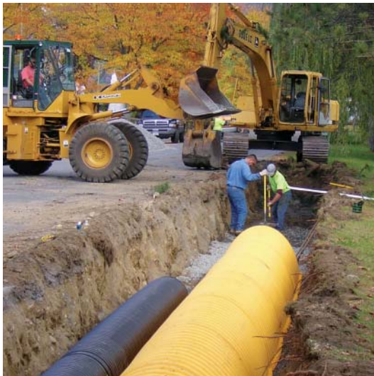
Installing stormwater treatment
