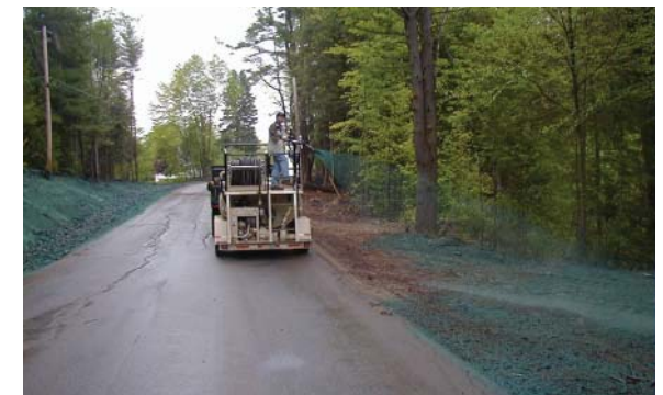
Hydroseeding road bank
