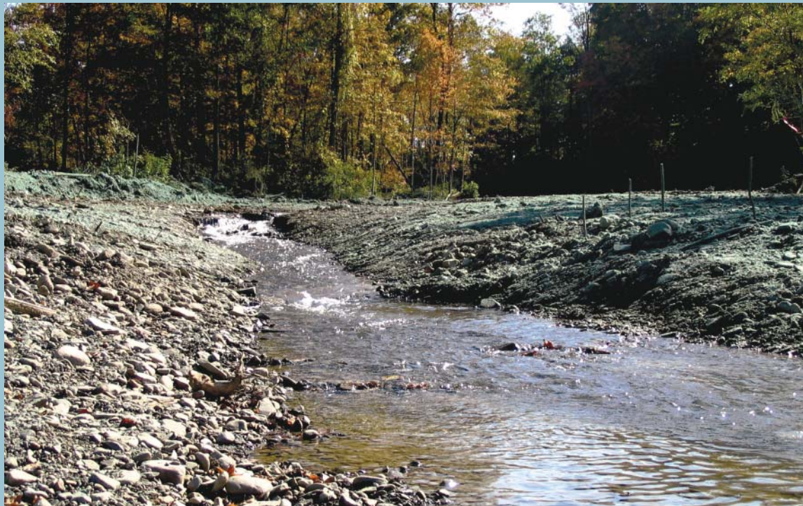
Six Mile Creek, streambank stabilization
