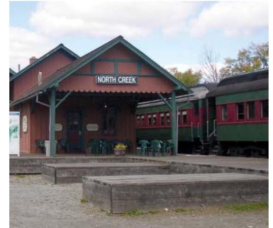
North Creek rail stop, North Creek
